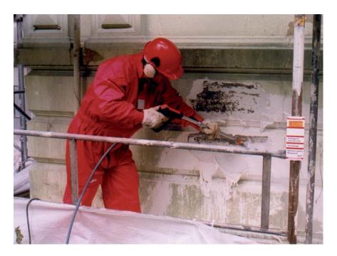
Old paint layers are removed in no time by means of the high-pressure and high heating power of OERTZEN POWERTRAILER.
